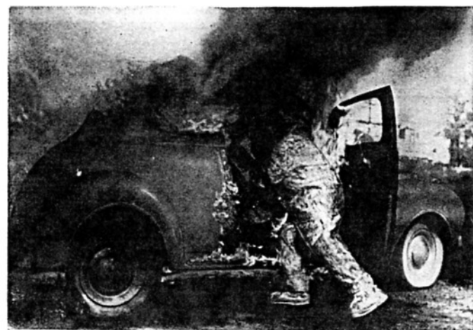
DEMONSTRATOR is unconcerned by roaring flames as he rescues dummy from behind wheel of auto. Flexible material is as light as ordinary suit and coat.
